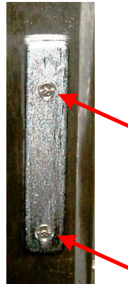
E) Remove the screws for strike plate and set aside, as these will be reused later.
