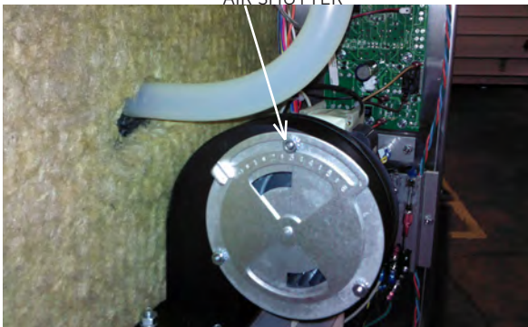
FIGURE 9 AIR SHUTTER
